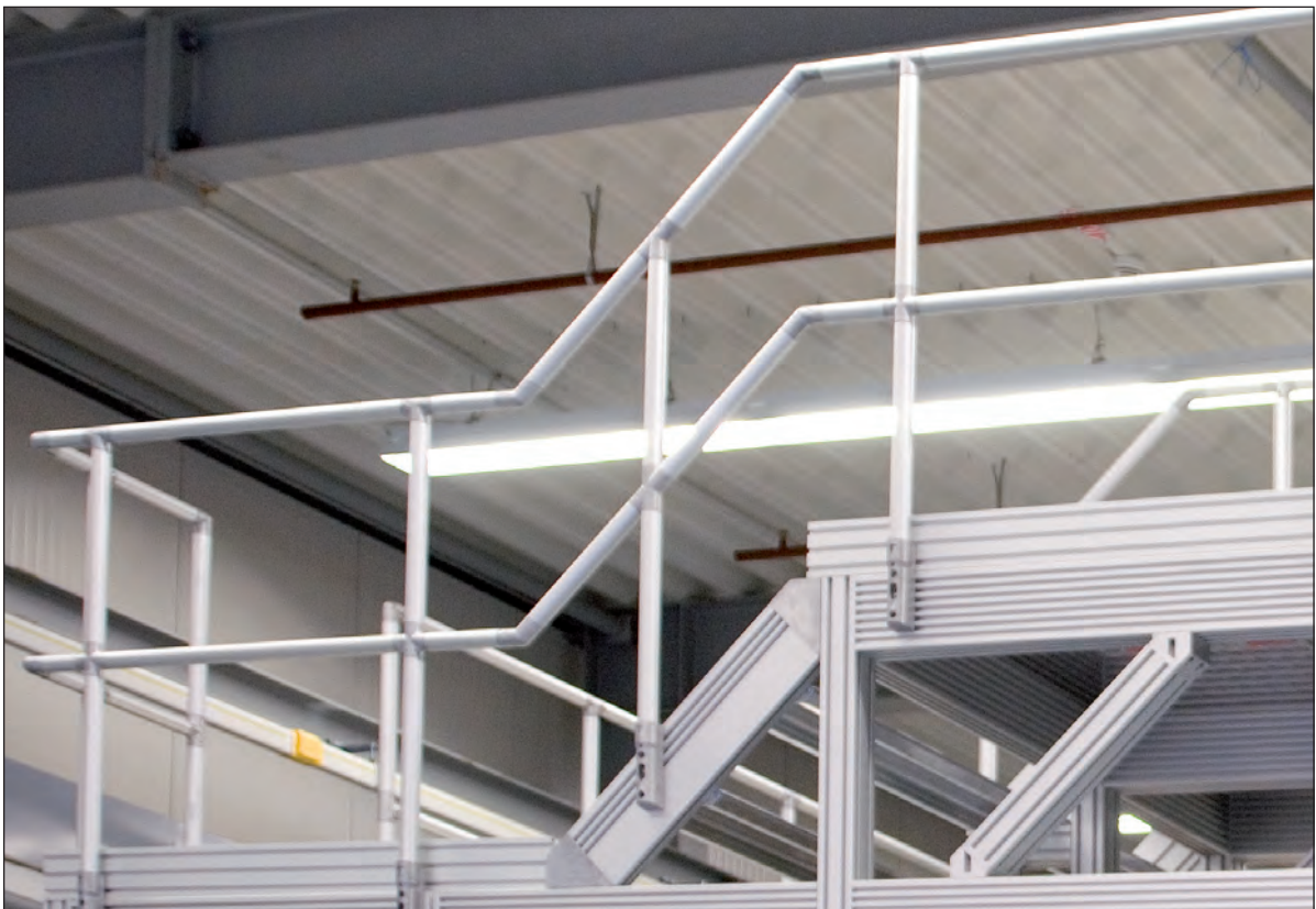
Staircase between two operating platforms.
