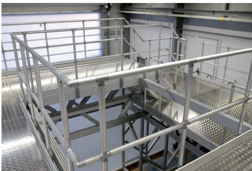
Working platform with ITAS railing
