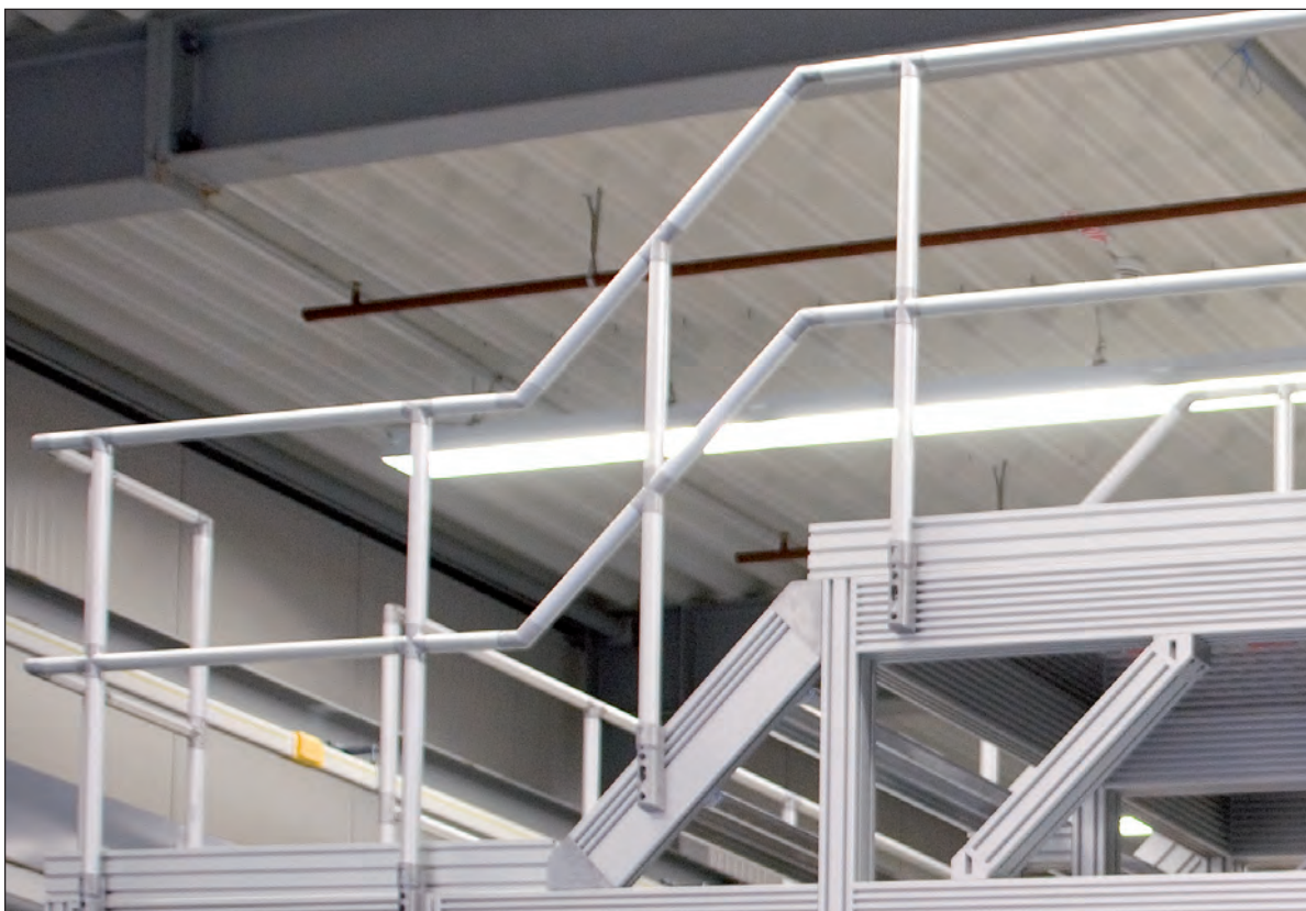
Staircase between two operating platforms.
